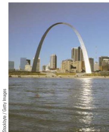
The Gateway Arch in St. Louis was designed using a hyperbolic cosine function (see Exercise 48).
